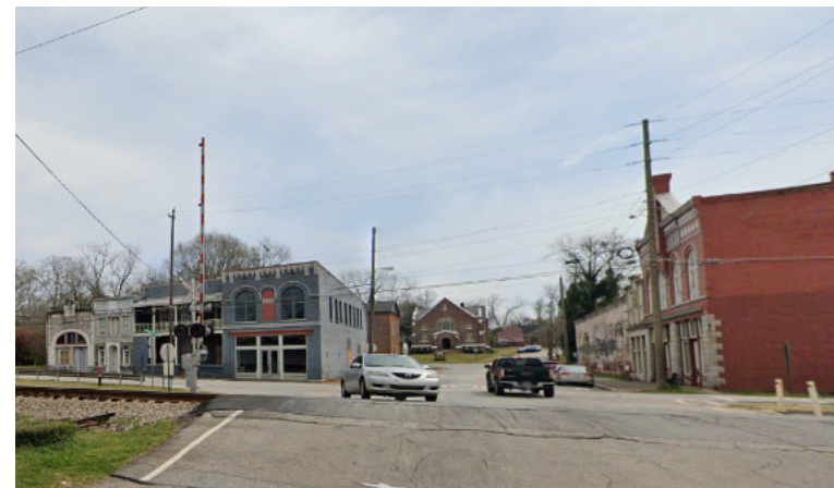
At-grade Railroad Crossing
